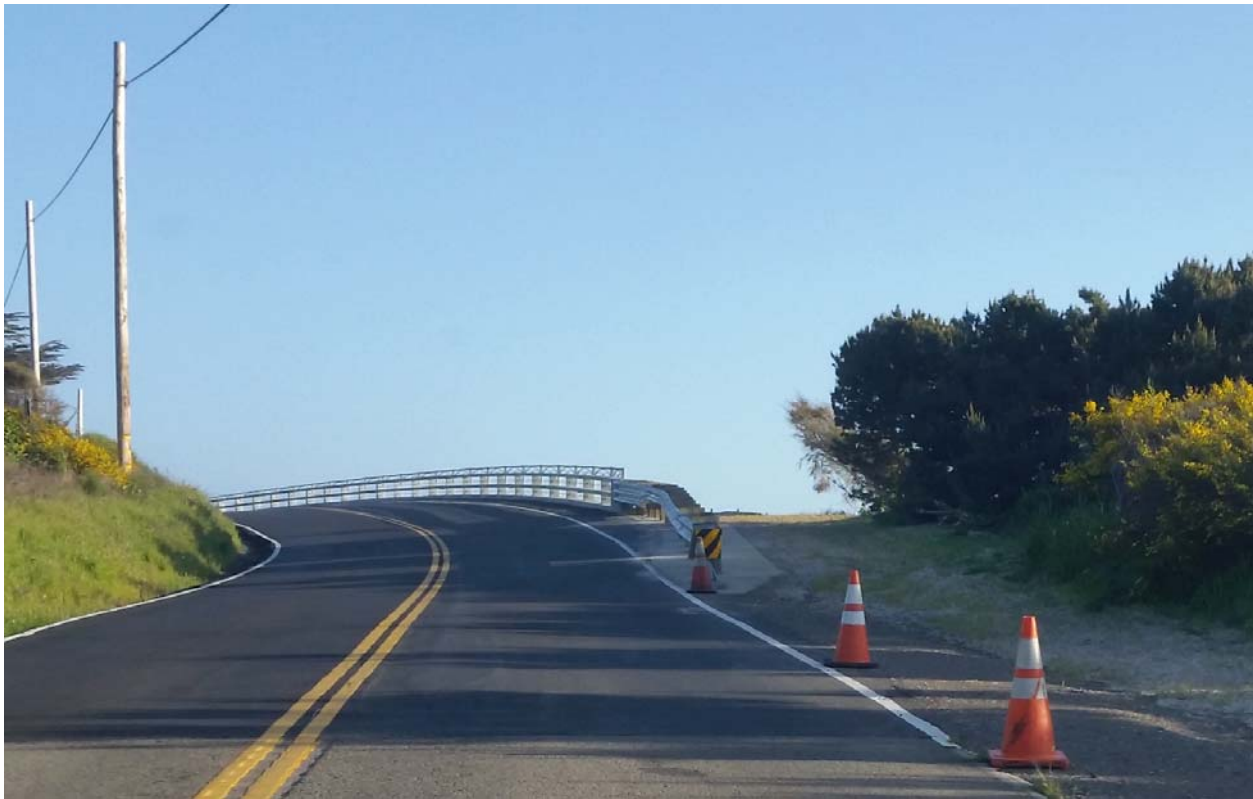
Approaching PM 78.8 on southbound MEN-001 showing guard rail posing a safety concern.
